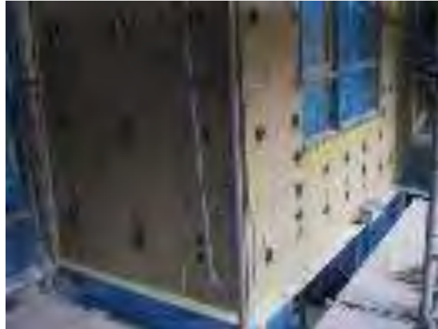
Post-Rehabilitation – Exterior Membrane & Fully Exterior Insulated
