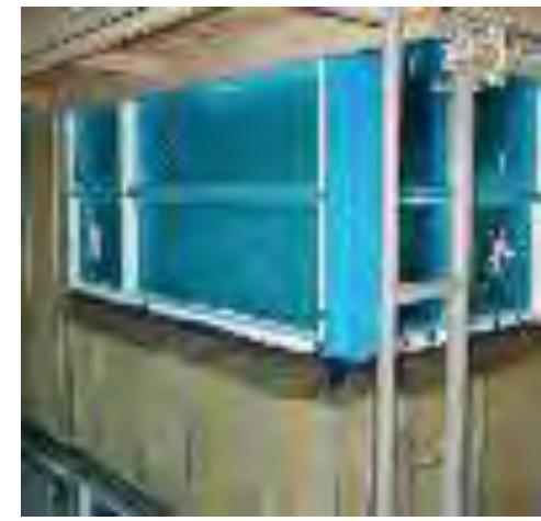
Post-Rehabilitation – Exterior Membrane & Fully Exterior Insulated
