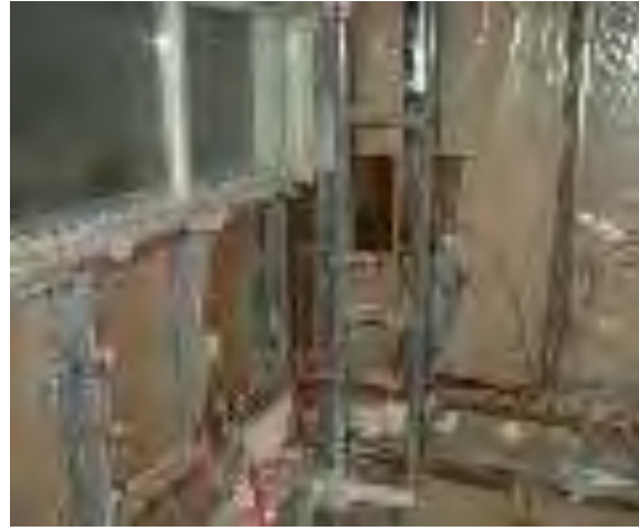
Pre-Rehabilitation – Stud Insulated, Lots of Thermal Bridging
