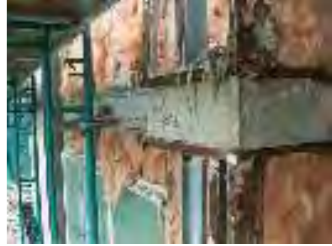
Pre-Rehabilitation – Stud Insulated, Lots of Thermal Bridging
