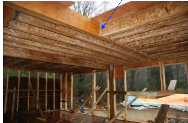
Wood I joists supported by LVL using galvanized steel hangers
