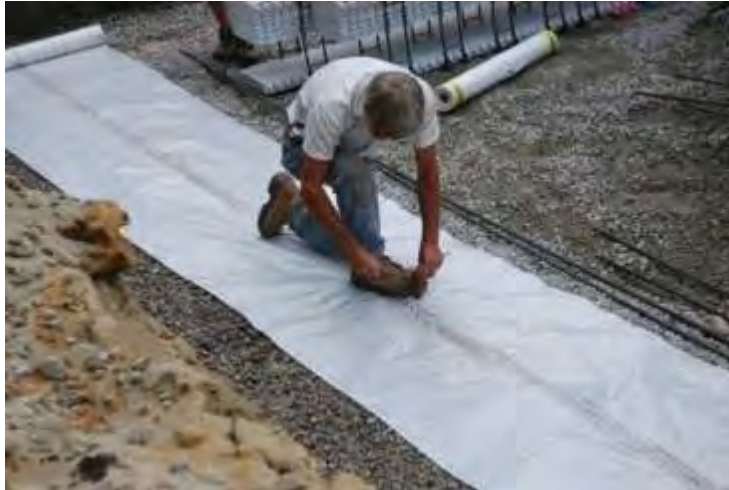
Monopour fabric footing laid out HD+C Ltd.
