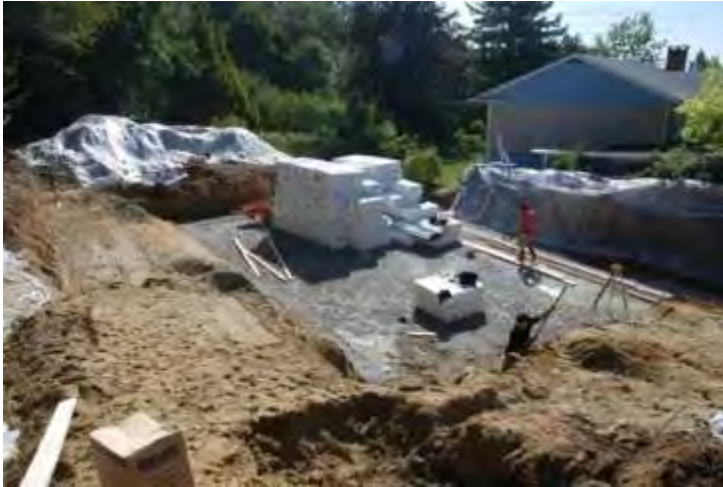
4" (100mm) thick gravel pad
