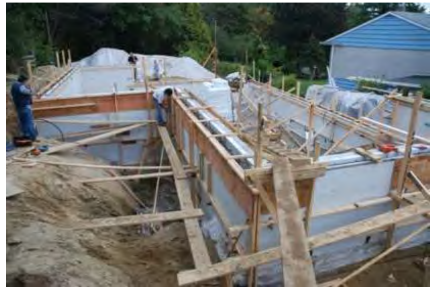
ICF wall bracing using 2x4's and plywood
