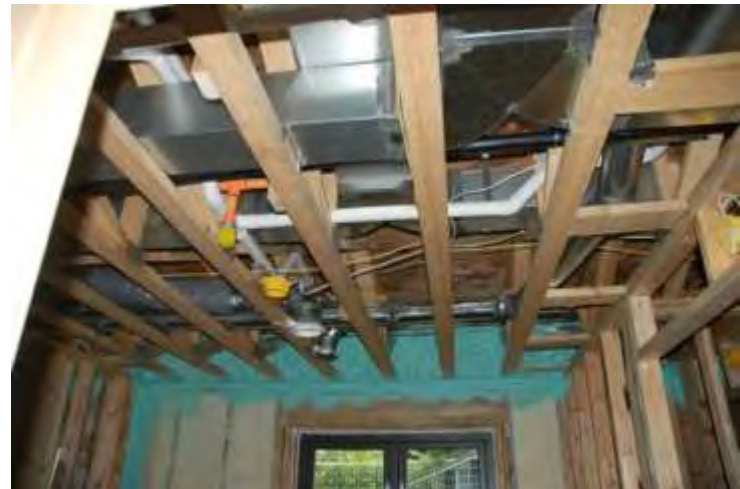
Heating, ventilation, plumbing and electrical services run through open web joists
