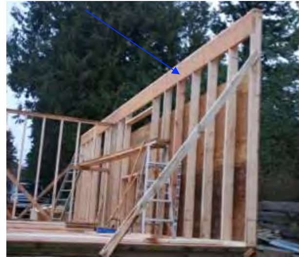
LVL let into top of studs to support floor joists and allow continuous insulation and eliminate window lintels
