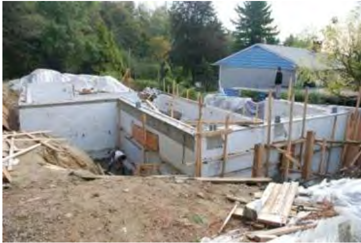
Concrete set and bracing removed
