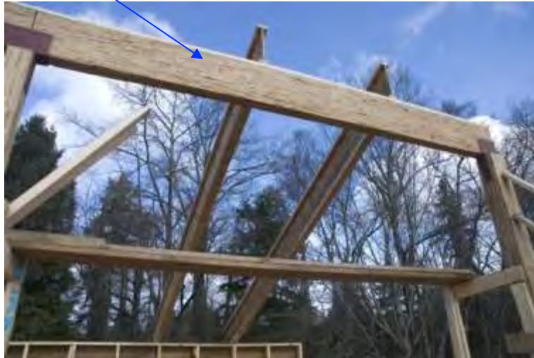
Central Parallam beam supporting wood I ceiling joists
