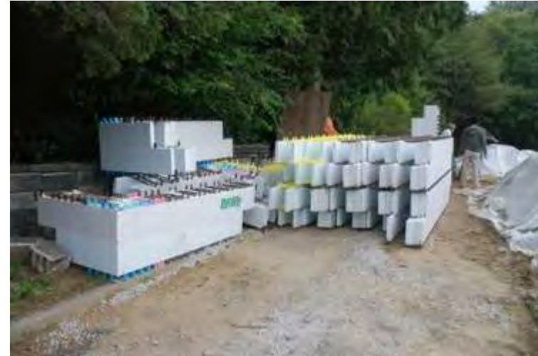
Bottom two rows of ICF prefabricated
