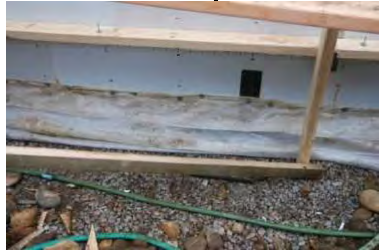
Fabric footing form screwed to ICF
