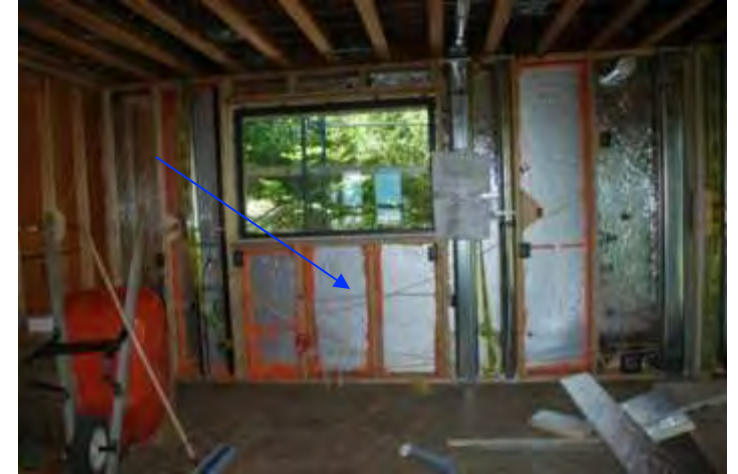
Vacuum insulation panels foamed in place
