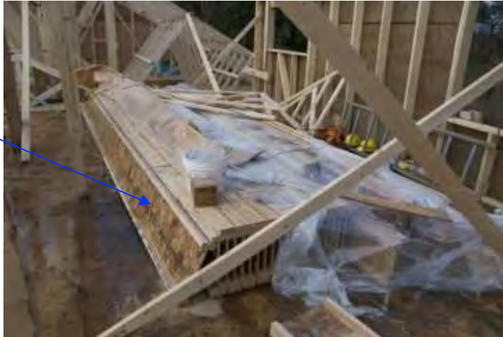
Wood I joists used for 2 nd floor framing
