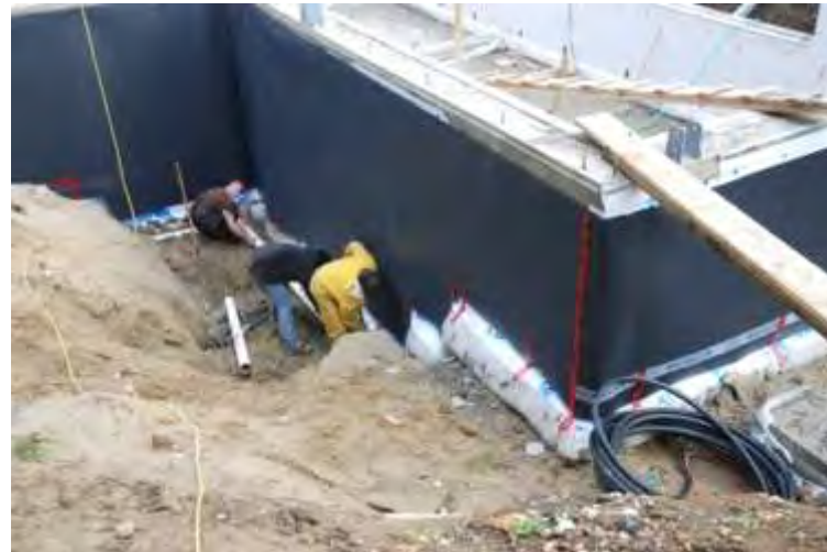
Waterproofing with plastic membrane and drainage mat drainage pipe run around footing and connected to sewer
