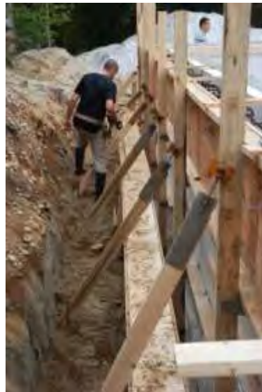
ICF wall bracing using 2x4's and plywood
