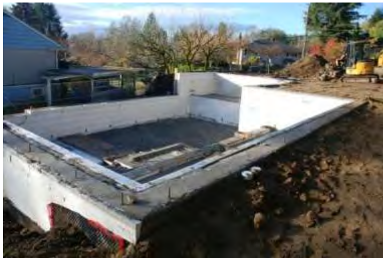
Foundation back filled HD+C Ltd.
