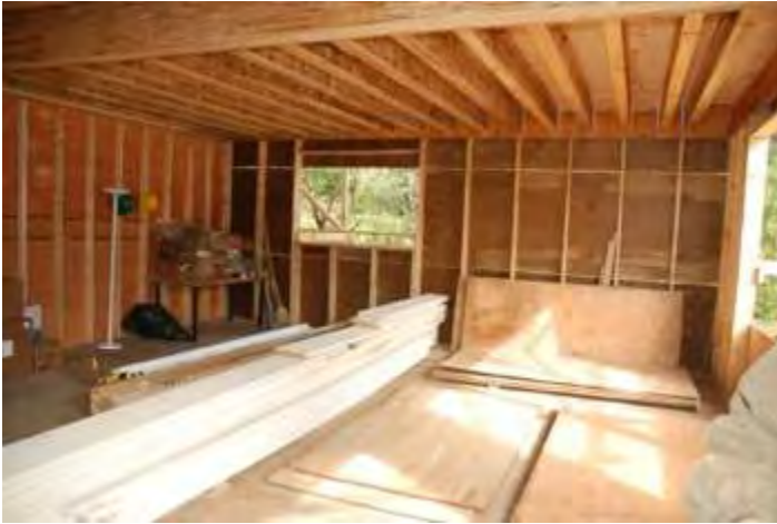
Exterior wall before insulation
