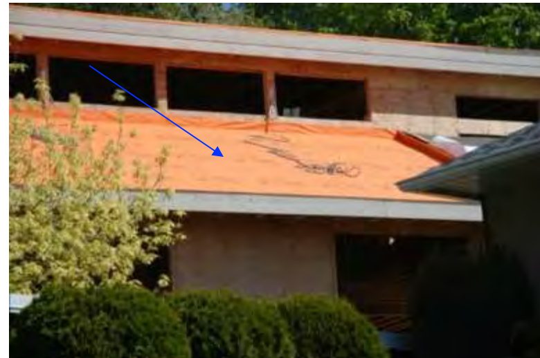
Vapour permeable water proof membrane
