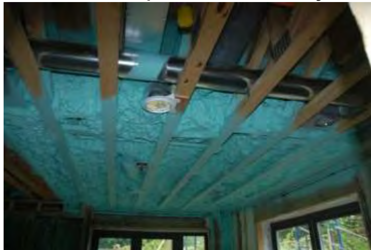
Allows for high insulation levels beneath solarium HD+C Ltd.
