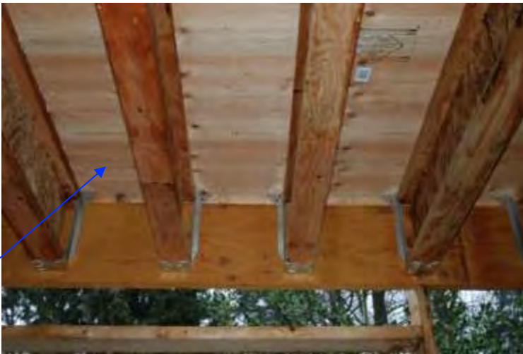
Floor sheathing \frac{3}{4} " (19mm) plywood HD+C Ltd.
