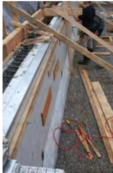
Concrete poured and vibrated
