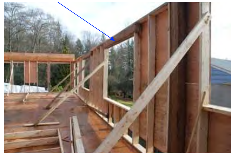
Parallam window lintels for large spans
