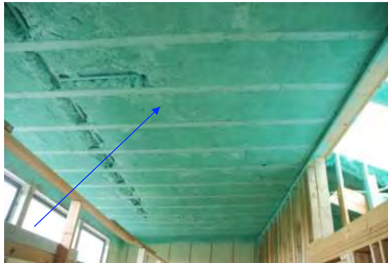
Upper roof cavities filled with castor bean oil based spray foam covered with vapour barrier paint
