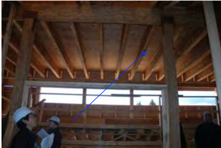
Upper roof showing joists and sheathing
