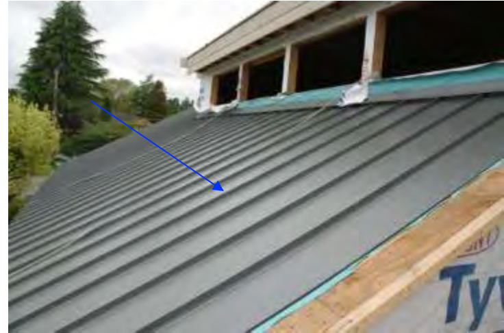
Standing seam sheet metal roof
