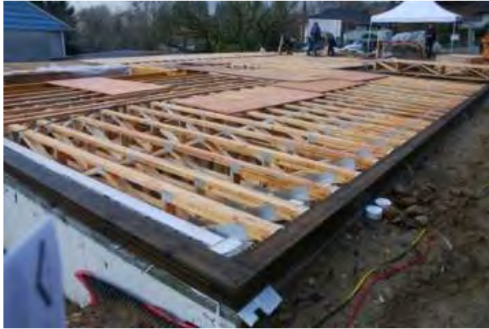
Main floor open web floor joists
