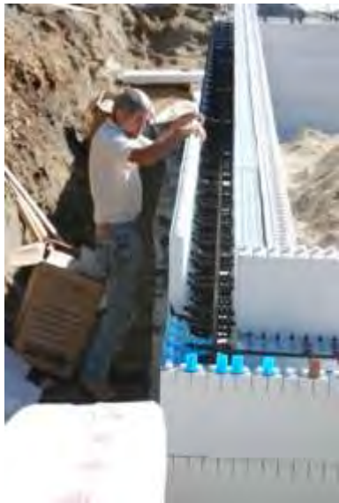
ICF wall assembled HD+C Ltd.
