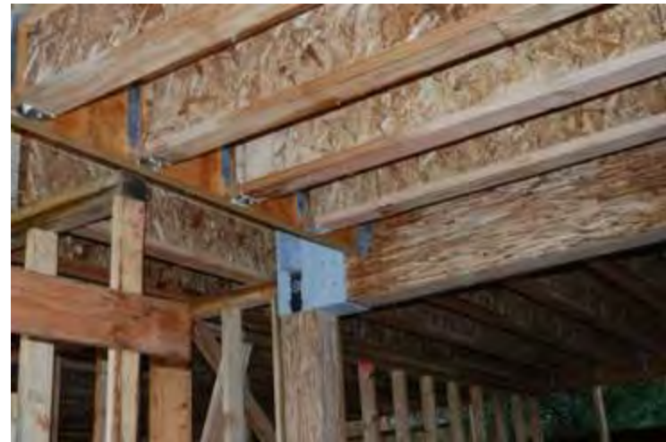
Wood I joists supported by LVL using galvanized steel hangers
