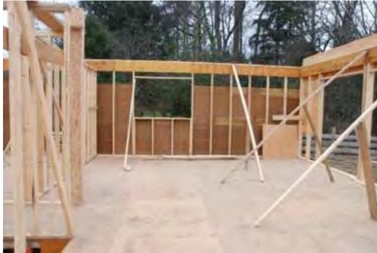
2x6 studs at 24" OC (610mm)
