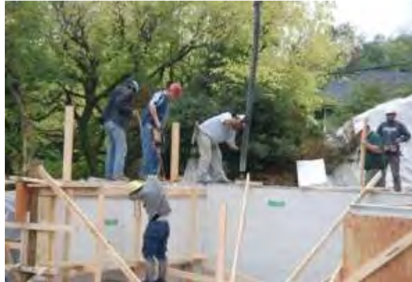
Concrete poured and vibrated
