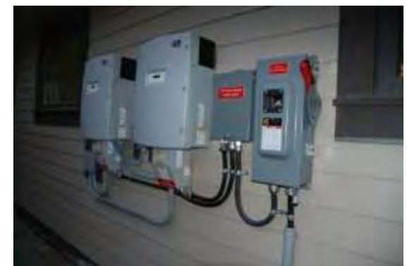
PV System Inverters
