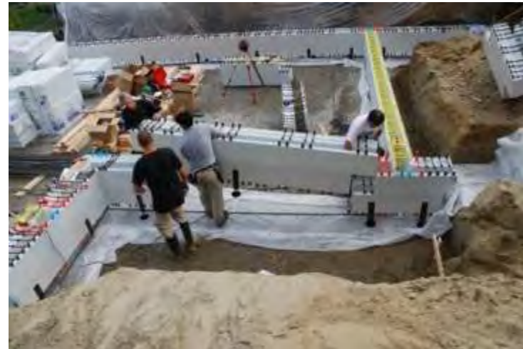
Bottom two rows of ICF prefabricated
