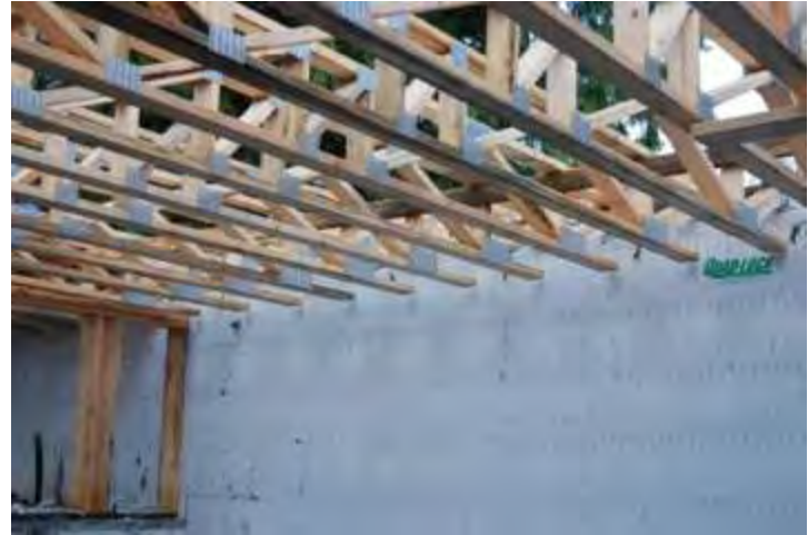
Open web floor joists from basement
