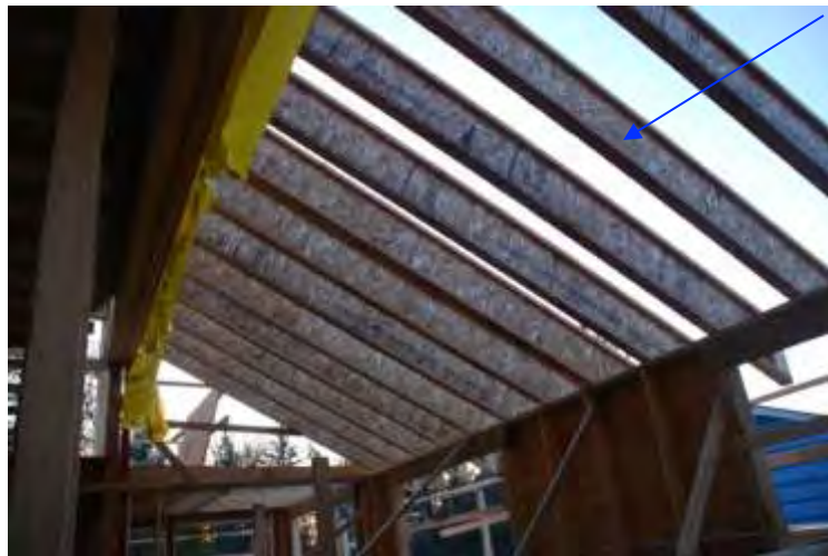
Wood I joists over living room HD+C Ltd.
