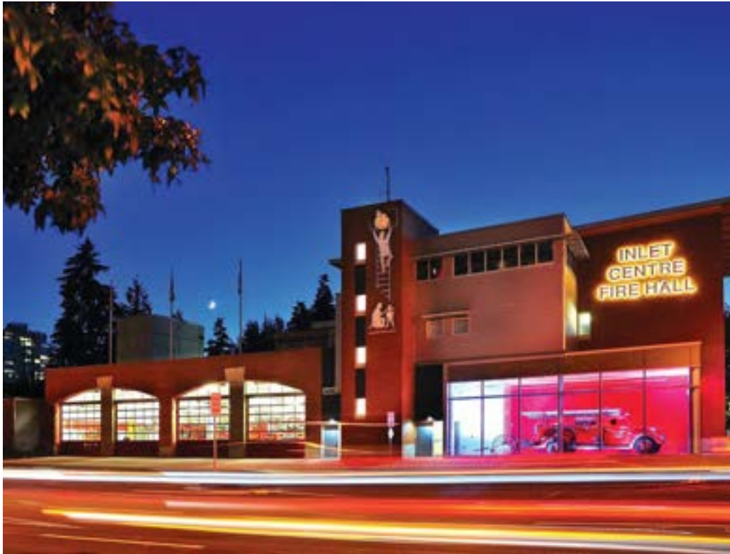
Inlet Fire Hall Port Moody
