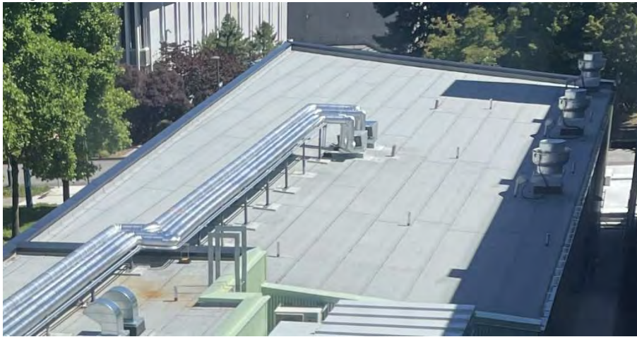
Roof with 11% slope on a sloped wood frame structure, clean appearance
