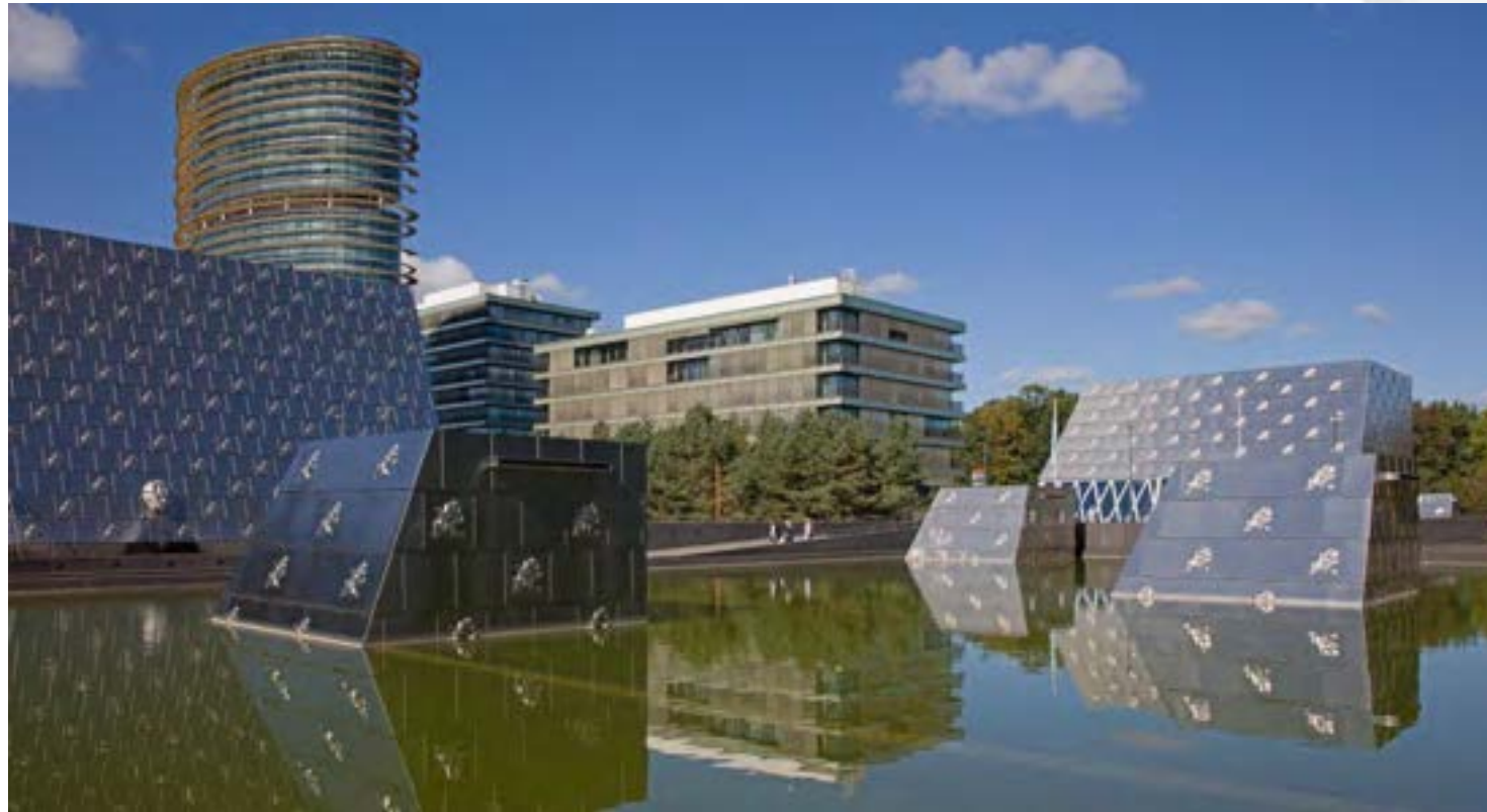
Water roof in Apeldoorn, Netherlands
