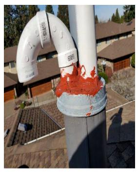
Occasionally the vents will be installed through a purpose-built roof flashing, but quite often they will be run up through the existing B-vent pipe. This can create a challenge regarding sealing multiple pipes.
