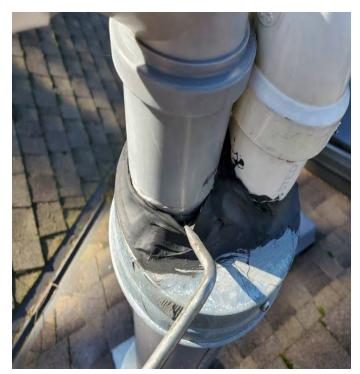
Some other clever ideas witnessed are to run the new exhaust through an existing vent. If the ducting is in the way, just disconnect it.
