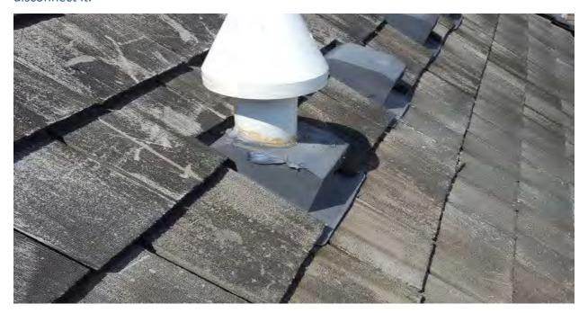
Here is another example where new exhaust pipes were run up through existing vents. The resourcefulness of the HVAC crews never ceases to amaze me.
