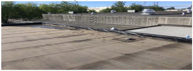
With concern, a call was made and we attended the site to review. The contactor was puzzled by the wrinkling and thought it was caused by internal pressures from within the building (basically an open warehouse).
