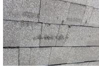
Scuff marks on asphalt shingles are quite common when the weather is warm. Some shingles are more resistant to scuffing than others. Most of the damage is a result of other trades working off of the lower roofs installing siding, windows, gutters or painting. Much of this damage occurs long after the roofing contractor has completed the work on that building.
