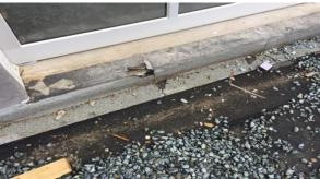
Damage to a completed membrane can also be caused from objects falling from above, or from concrete forms built over a completed waterproofing membrane. While this damage is large and clearly visible, other damage noted in this area was small and barely visible. (Upper Left)
