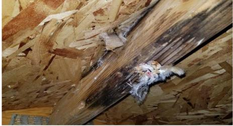
Eventually the fabric itself will start to rot. In this case, the strap was cut in the attic but left on the roof. It should be very clear the danger that this strap poses at the roof level.
