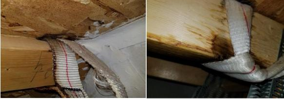
Attic reviews reveal that when fabric anchors are left in place, the moisture is drawn up into the attic through the fabric & starts to decay the roof framing and sheathing. Mold has been observed in these locations as well.
