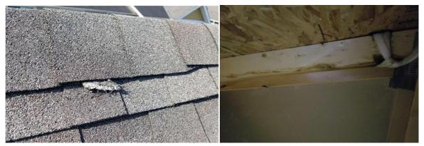
When the roof anchor is left in place, this allows it to absorb water and draw the water through capillary action into the attic space.
