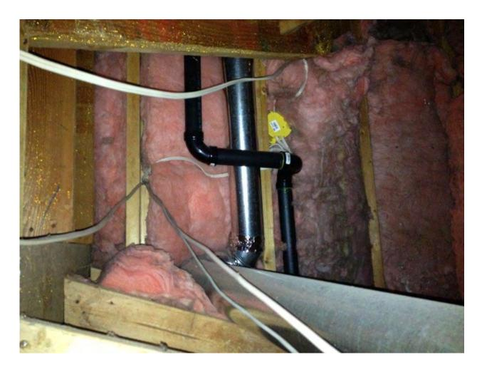
The solution was to secure the pipe in the attic, preventing it from dropping. Testing the pipe by applying light pressure downwards or accessing the attic during the roof replacement will allow you to take action to prevent this problem from re-occurring.
