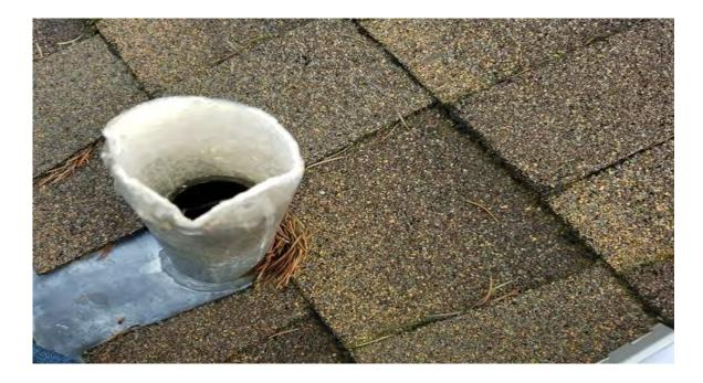
Accessing the attic revealed a long vertical pipe connected to an elbow turning the vertical pipe to horizontal, where it traveled another 4' before turning down and disappearing through the attic floor. This horizontal pipe was originally 18" up from the attic floor. Over time this pipe sagged, as it was no longer being held at the roof level by the rubber seal on the old plastic plumbing flashing.
