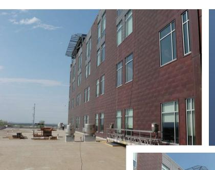
The cladding for the project consisted of copper and zinc cladding over framing and insulation
