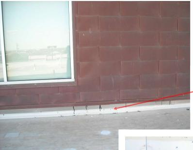
Copper creates high heat, especially on south-facing elevations. The liquid asphaltic dampproofing was exhibiting signs of melting and breakdown
