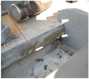
The zinc flashing at the top of the columns (and helipad connections) acted as funnel for water to enter into the cavity behind the metal cladding
