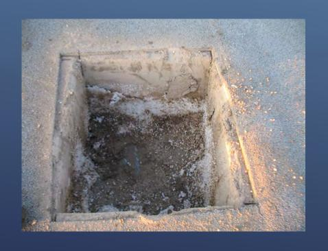
Moisture accumulation was evident at the interface of the deck and the insulating concrete.
