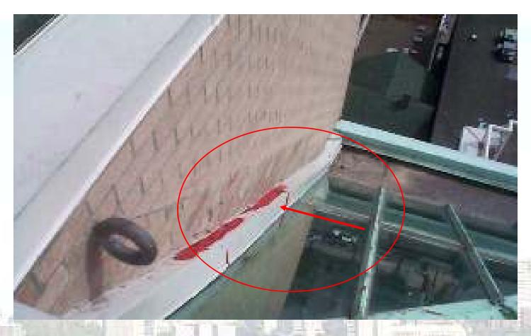
Dumb-sloping a flashing toward a wall AND not realizing that the horizontal coupler of the skylight is the cause of the leak
